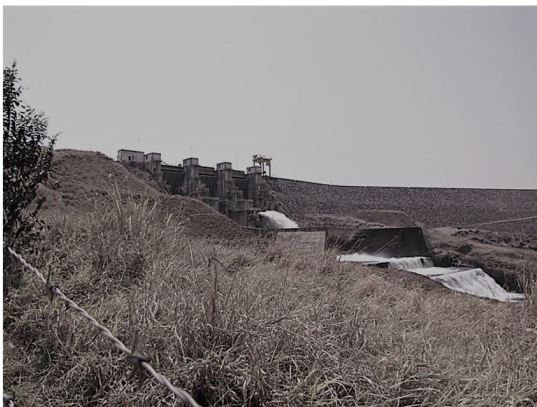
Figure 3. Capim Branco HPP: closed pourer and flow operation using valve opening. Source: Tarcísio Castro (Personal Archive).
