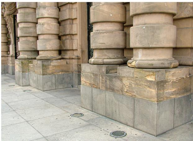
**Figure 1.** Degradation of the Itararé Sandstone in the front facade of the Municipal Theater of São Paulo.
