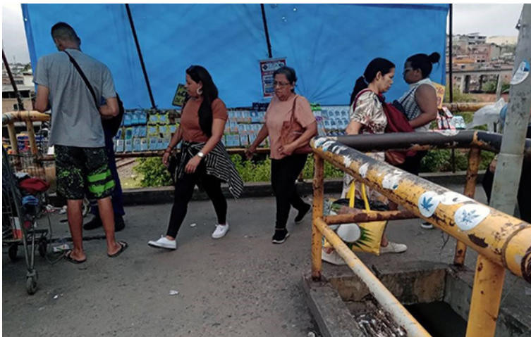
Figure 4 – Photo of the walkway leading to the Pavuna metro station, showing an informal sales counter using the metal railing of the ramp as support. On the right we see a metal bar pre-fixed to the metal railing of the ramp, ready to serve as a support
